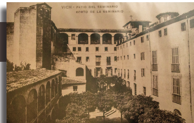
Courtyard of the former seminary of Vic
